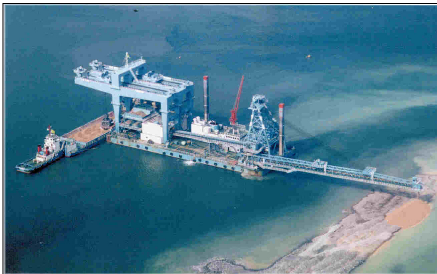
Figure 3: Grab bucket reclaimer.
